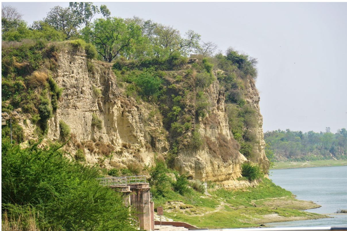
Image 44 : Erosion Prone Bank At Manikpur
